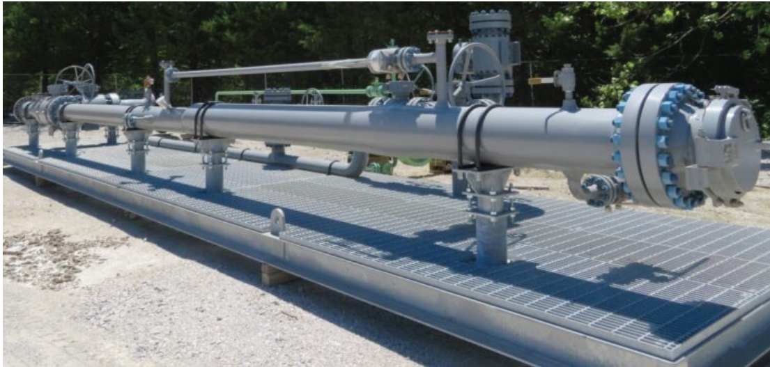
Figure 2. Pipeline trap.
