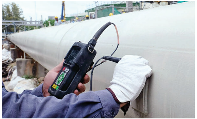
Figure 7. Measuring wall thickness.
